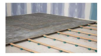
When using battens for an increased airspace, no fixings should be screwed into the pad or the perimeter, and battens must be at least the width of the pad, as shown.
