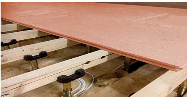
Resilient Saddle Headcap & Pedestal Assembly with Smartspan calcium sulphate overlay
