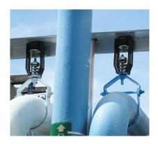
Isolation hangers shall be selected by the manufacturer for each specific application to comply with deflection requirements as shown on the Vibration Isolation Schedule or as indicated on the project documents.
